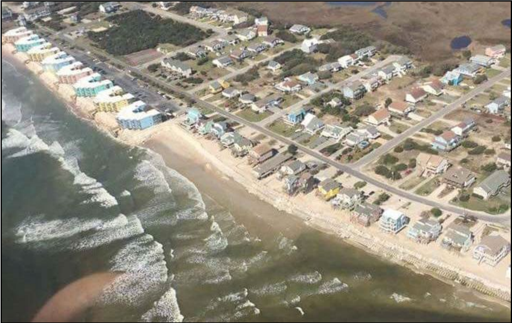
Figure 2-3. Threatened structures along NTB north end shoreline - March 2016 aerial imagery
