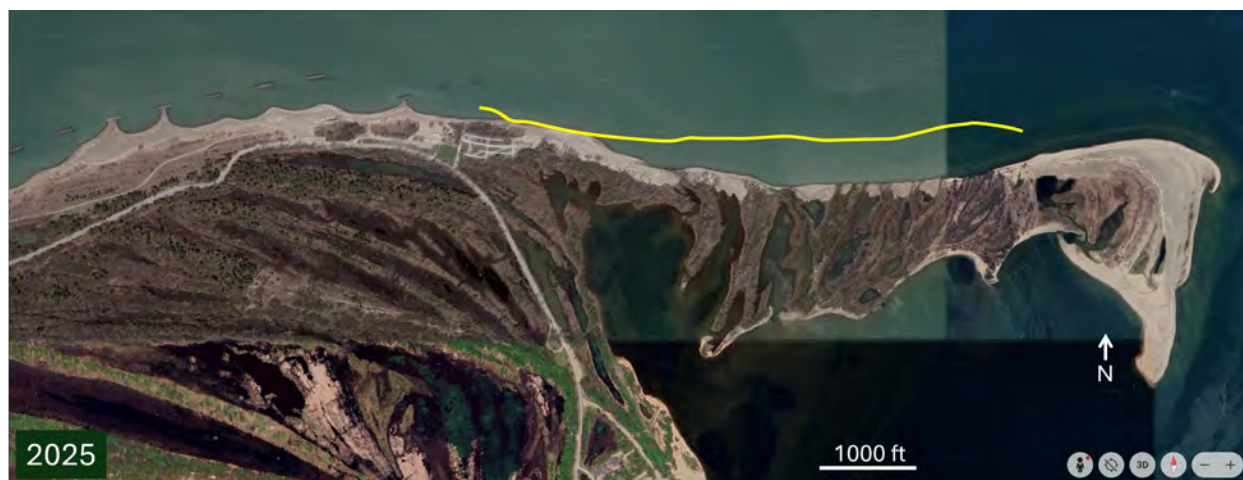
Figure 11. Presque Isle in 2006, 2016 and 2025 (top to bottom), showing continued, progressive erosion along the eastern end of the peninsula, downdrift of the field of breakwaters (Google Earth). The yellow curve in each image shows the shoreline position in 2006.
