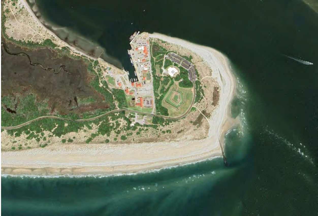
Figure 8. The terminal groin at the East end of Bogue Banks, and Fort Macon, NC in 2023.
