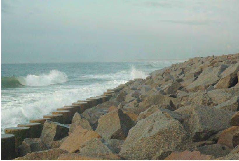
Figure 4. South end of the Fort Fisher revetment.
