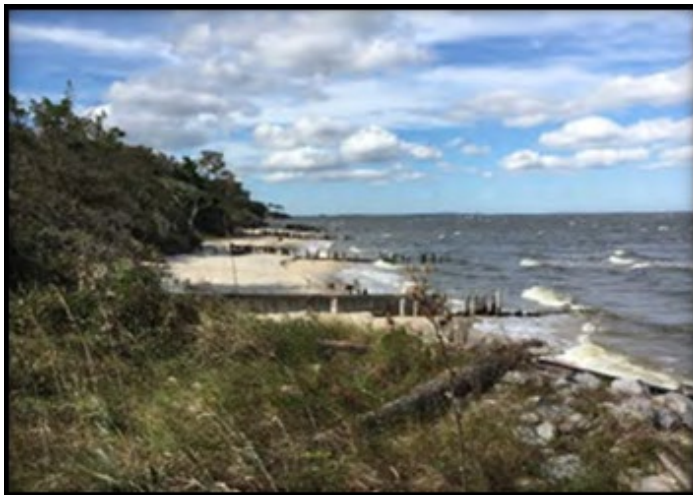
Damaged wooden groins installed along a section of shoreline.
