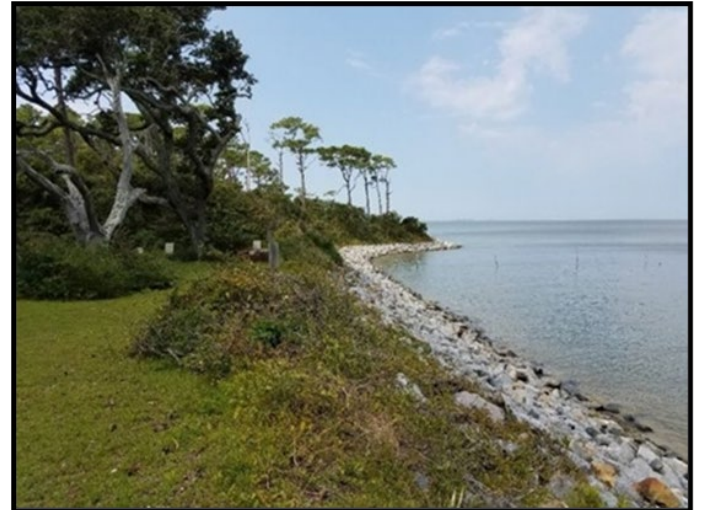
Rock revetment installed along Dough Cemetery shoreline.
