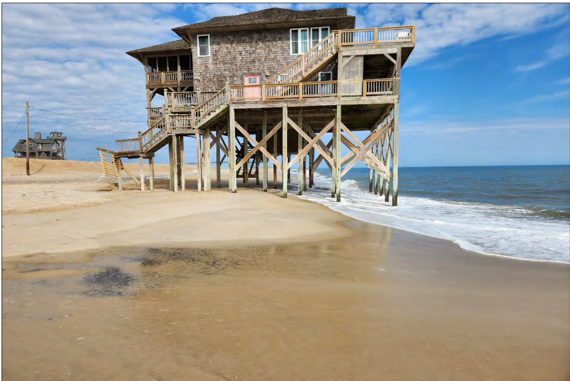
FIGURE 1.2b. Beach conditions along the Rodanthe reach offer little to no storm protection for many first-row homes, with several properties on the intertidal wet beach. The recent collapse of multiple such properties has compelled the County to investigate sand needs for a nourishment project at Rodanthe. The ground photo location is marked in the upper photo with a red circle.
