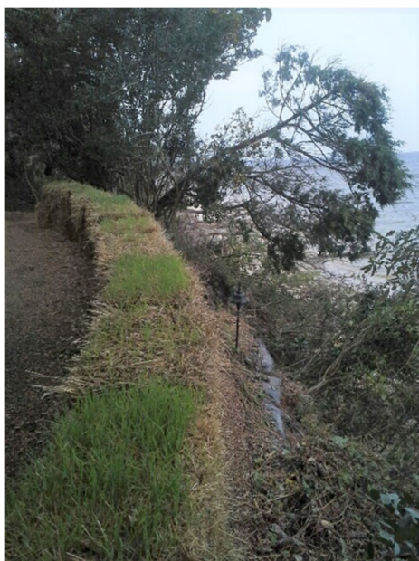
Eroding bluff of the Elizabethan Gardens.
