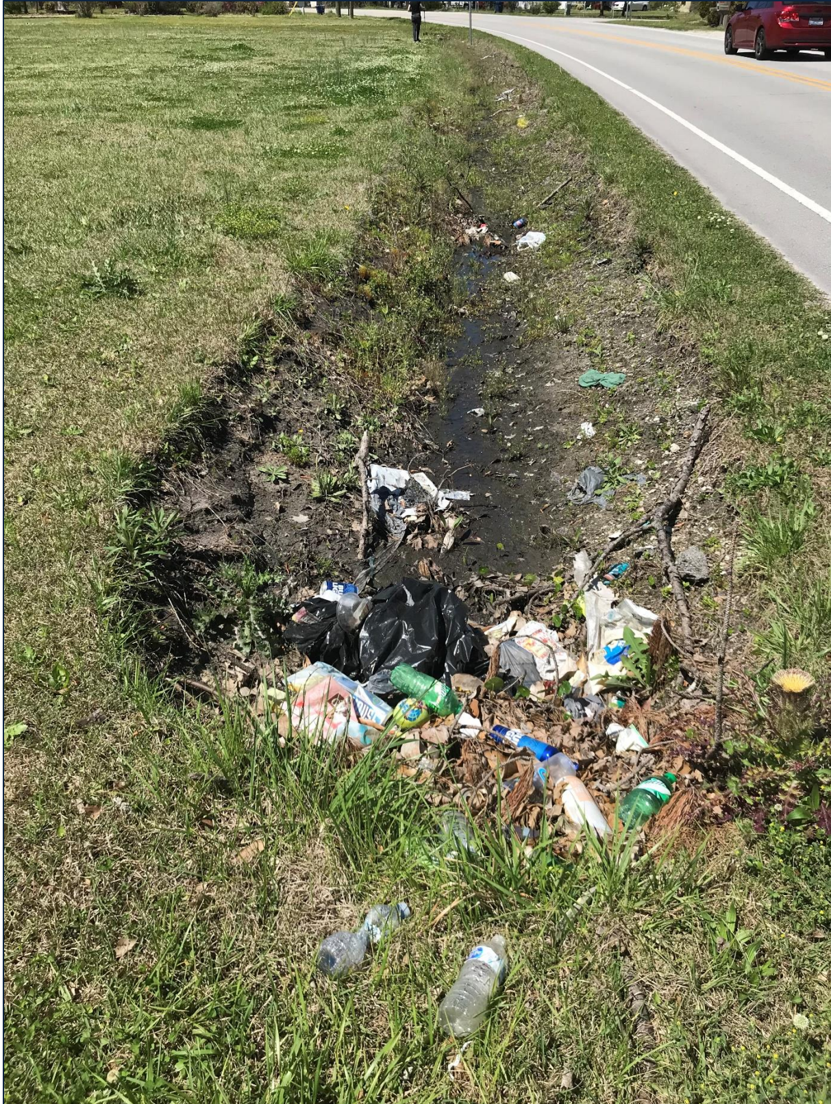
Figure 14 - Litter in Ditch at H-3
